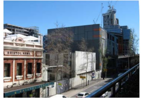
Figure 2.1 The subject site is between the Bristol Arms Hotel on the left and the City North Substation on the right. Note the utilitarian structures on the subject site
