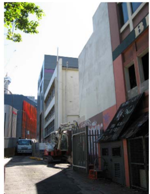
Figure 2.2 The vacant parcel of land on the western boundary, with the Bristol Arms Hotel on the right. Note the Substation behind the three storey building currently on the subject site. The Western Distributor is to the left
