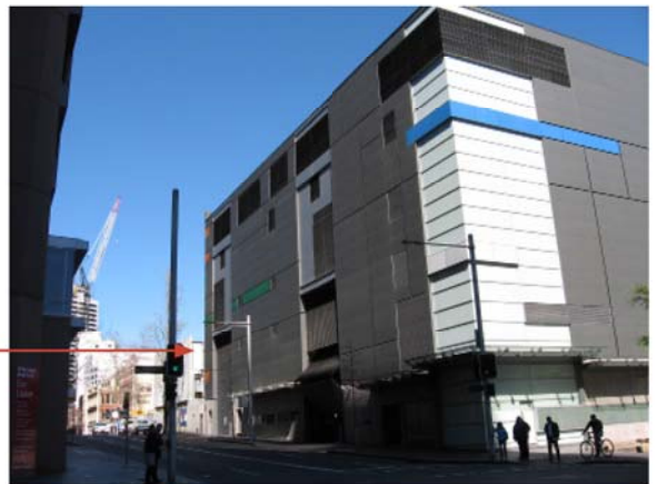
Figure 2.8 Western side of Sussex Street on the corner with Erskine Street, with the Substation on the right, next to the subject site
