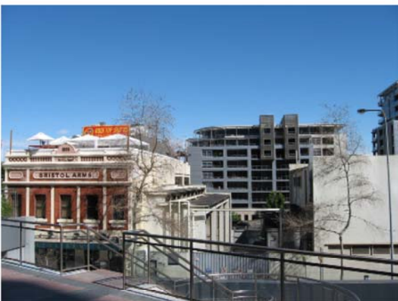
Figure 2.9 Looking across Sussex Street to the subject site, with the Shelley Street apartments beyond. Note the Bristol Arms Hotel on the left
