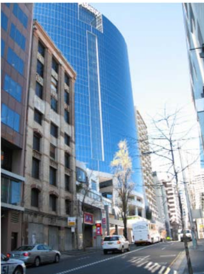
Figure 2.7 Eastern side of Sussex Street with the glazed commercial tower opposite the subject site
