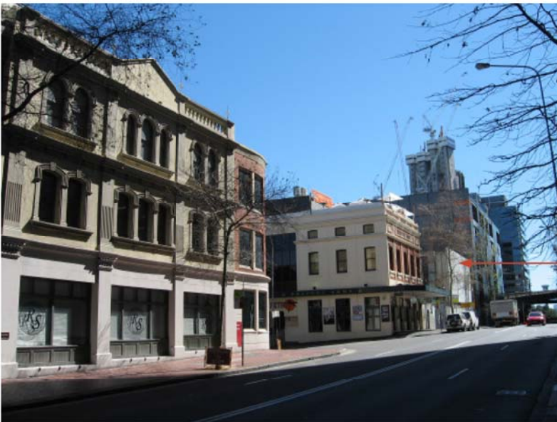
Subject site at 65-79 Sussex Street
